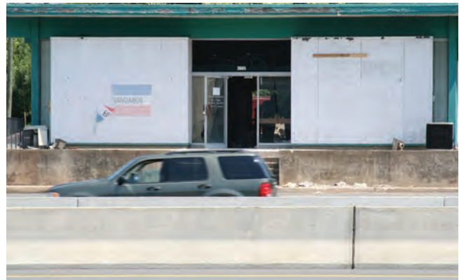
Access management limiting accessibility to businesses.
